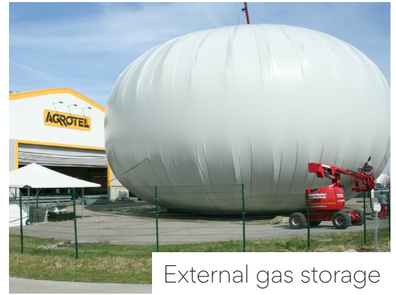
Double membrane gas storage
